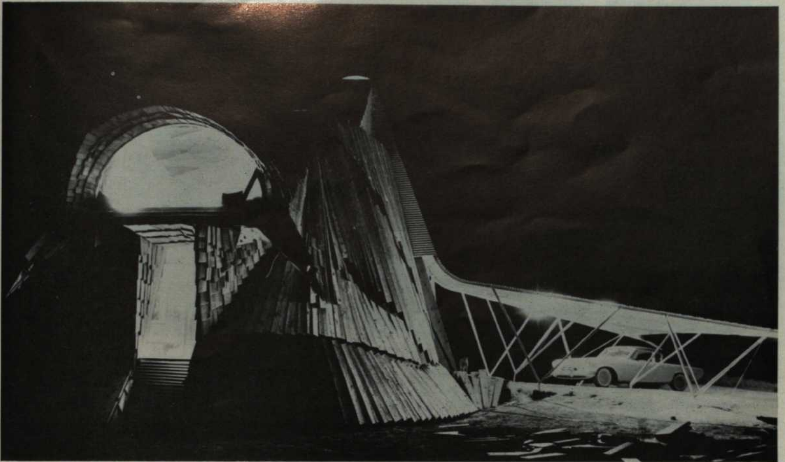
The Greene House at night is a startling sight with light streaming from its mushroom-shaped windows and accenting the corrugated aluminum.
